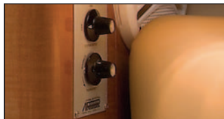
AIR CONDITIONING 5,000 BTU R265
